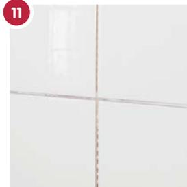
11 After the adhesive has set, remove horizontal and vertical battens.
