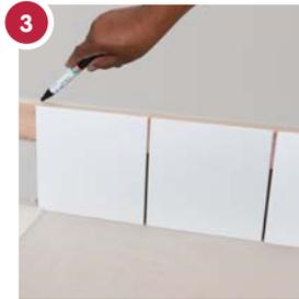
3 Set out a row of tiles across the wall over the batten and adjust so that equal cuts at least half a tile wide will be made in each corner. Mark the batten where the first tile will be placed. Remember to leave room for tile spacers.
