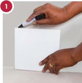
1 Find the lowest point on the floor line and mark the wall one tile high from the floor at this point.
