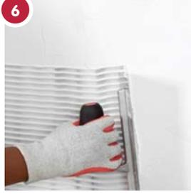
6 In a horizontal direction, notch the adhesive with the notched wall trowel or wall applicator. Do not spread more adhesive than can be tiled onto in approximately 15 minutes.
