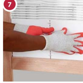
7 Using dry tiles, begin in the corner of the battens placing tiles horizontally. Tile spacers ensure even joints between tiles. Remove before grouting. Leave cut tiles until last.
