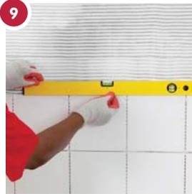
9 Check tiling regularly with a spirit level to ensure that horizontal fixing is being maintained.
