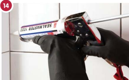
14 Provide movement joints in all horizontal and vertical corners. In large areas keep these approximately 5m apart. Rake out joints and leave ungrouted. Fill with TAL Goldstar Sealmaster 1000 polyurethane joint sealant.
