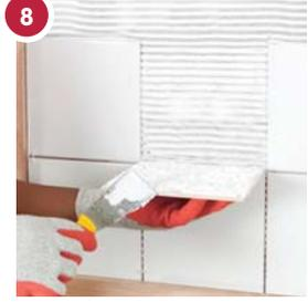
8 Bed the tiles in firmly using a rubber mallet. Remove the occasional tile to check that good contact with the adhesive is being made.
