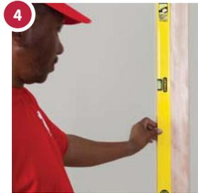
4 Nail a vertical batten to the wall so that the inside edge of the batten coincides with the mark for the first tile. Check with a spirit level to ensure that the batten is perfectly vertical.
