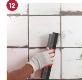
12 Allow adhesive to dry before grouting. Use TAL Wall and Floor Grout, available in a variety of colours. Work grout well into joints with a rubber squeegee.
