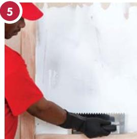
5 Use the appropriate TAL tile adhesive, like TAL Flex, and commencing in this corner, spread the adhesive onto the wall with the straight edge of a notched wall trowel or wall applicator.
