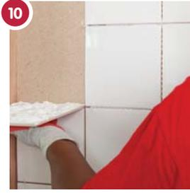
10 Measure and cut each tile required to fill in corners and bottom row, leaving room for tile spacers. Butter the back of the tile with adhesive, place cut edge into the corner and press firmly into place.
