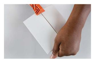
Use a tile breaker to apply pressure on the scored tile to achieve a clean break. Use a tile grate to neaten the cut area.
