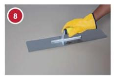
Spread the mix using a 600mm extended straight-edge steel trowel and work to a smooth, level surface. Trowel marks and high spots can be removed with coarse sandpaper or a corundum stone when the screed is dry.
