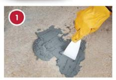
All "lows" and voids in the floor must be identified and cleaned out, and must be filled with TAL Rapidfix prior to applying TAL Superscreed, and all "highs" or trowel marks must be identified and ground down. All defective areas of concrete/screed must be removed and made good using TAL Rapidfix.
