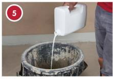
TAL Screedbinder should replace the water in the mix when TAL Superscreed is applied in high traffic areas, all exterior or exposed areas, wet areas, where building movement is expected, and where thermal expansion and contraction is expected (ie under-tile heating).
