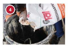
Add 20kg TAL Superscreed to 5 litres of clean, cool water while stirring and mix until a smooth, lump-free paste is obtained. Mechanical mixing is essential for good mixing and uniform dispersion of product. For best results use a full bag in one mix.
