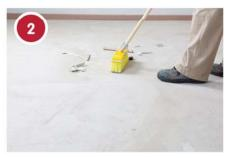
The substrate to be screeded must be in good condition, structurally sound, and free from all traces of contamination such as curing and sealing compounds, grease, grime, old floor coverings, fixatives, paint, etc. The floor must be swept to remove all traces of dust and loose particles. (Vacuuming is preferred.)
