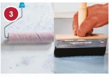
NOTE: All surface beds must have a damp proof membrane, and the substrate must have a moisture content of 5% or less before TAL Superscreed can be applied.
