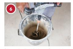
Stir occasionally whilst in use. Do not mix more than can be used in 20 - 30 minutes. Never add more liquid to a mix which has been left standing for too long, as this will compromise the integrity of the screed. Warm weather may shorten the working time of the mixture. Extreme cold conditions will affect the setting time of the screed.
