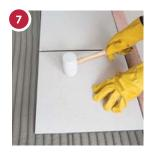
Use dry tiles. Butter the back of heavily ribbed tiles. Bed the tiles firmly into the adhesive using a rubber mallet.
