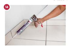
Provide movement joints in all corners. In large tiled areas keep these approximately 5m apart internally and 3m apart externally. Rake out joints and leave ungrouted. Fill with TAL Goldstar Sealmaster 1000 polyurathene joint sealant.
