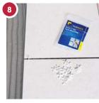
Use tile spacers to create uniform spacing. Remove before grouting. Never butt ceramic tiles hard up against each other.
