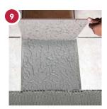
Lift the occasional tile to check for full coverage of adhesive on the back of the tile. No voids should occur underneath the tiles.
