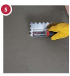
Start at the centre of the room. Use the appropriate TAL adhesive, like TAL Goldstar 6, and with the straight edge of a floor trowel, spread the adhesive onto the floor.
