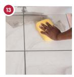
Remove the excess grout with a sponge. Allow the grout to dry and then polish with a dry cloth.
