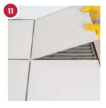
Measure and cut each tile to fill edges leaving room for the tile spacers. Butter the back of the tile with adhesive, place the cut edge towards the wall and bed firmly into place using a rubber mallet.
