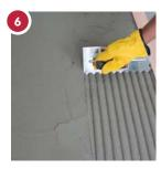
In a horizontal direction, notch the adhesive with the floor trowel or floor applicator. Do not spread more adhesive than can be tiled onto in approximately 15 minutes.
