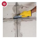
Allow the adhesive to dry before grouting. Use TAL Wall and Floor Grout or TAL Quarry Grout available in a variety of colours. Work grout well into joints with a rubber squeegee.
