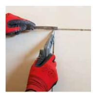
**STEP 3 Remove existing grout.** Rub the toothed blade of the grout rake back and forth until it has worn away the grout
