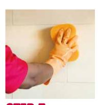
STEP 7 Clean off excess grout Wait 2-6 hours then wipe away excess grout with a damp sponge Tip: clean tools before the grout hardens
