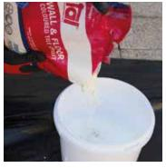
**STEP 5 Mix the grout** Follow the packaging instructions and if you are grouting a wet area, like a shower, replace the water in the grout mix with TAL Bond
