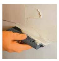
**STEP 6** Apply Grout Use a grout squeegee and fill the joints completely
