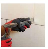
**STEP 4** Clean up the edges using a small chisel and hammer Tip: ensure you don't chip the adjacent tiles
