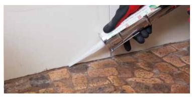
**STEP 9** Seal the perimeter joints in the shower with a silicon sealer
