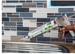
Apply a silicone sealant into the perimeter joint between the mosaics and counter top and in any corners
