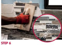
Firmly bed the mosaic sheets into the adhesive using a wooden beating block or a grout float to keep them level. Allow the TAL Mosaicfix to squeeze through the grout joints to form the grout
