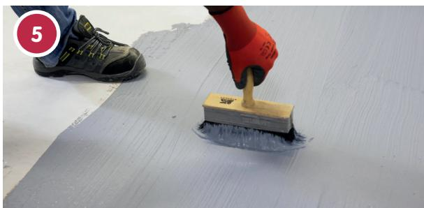
Using a builders block brush apply the TAL Keymix & TAL Keycoat slurry to the surface, ensuring good coverage, ie. the slurry coat must fully cover the substrate.
