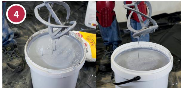
Using a mechanical mixer, mix well. The slurry must have a smooth, paint-like consistency.
