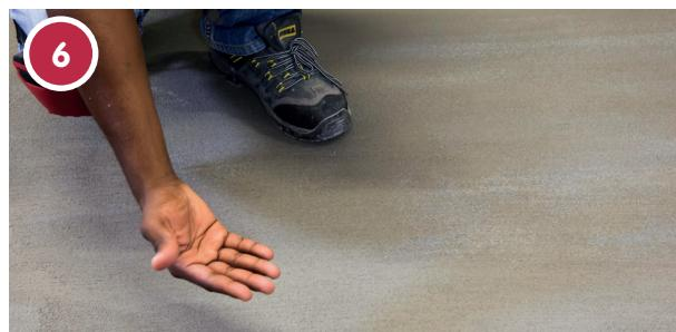
Allow to dry between 1-2 hours and check that it is touch-dry before commencing tiling.
