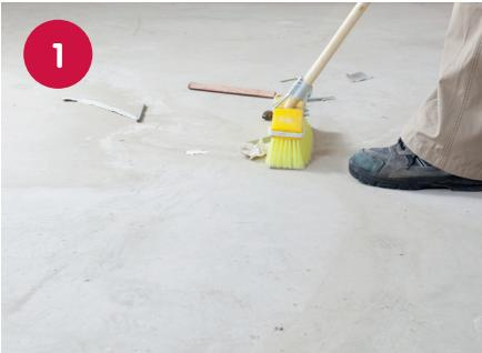
The substrate to be waterproofed must be clean, dry, firm and sound free from dust, loose particles and surface contaminants, and must have a moisture content of less than 3% before the waterproofing can be applied.
