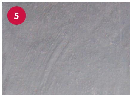
For the main area application apply a coat of TAL Superflex over the primed surface. Immediately bed the TAL Superflex Membrane into the wet TAL Superflex, ensuring there are no wrinkles in the membrane and no air pockets trapped underneath.
