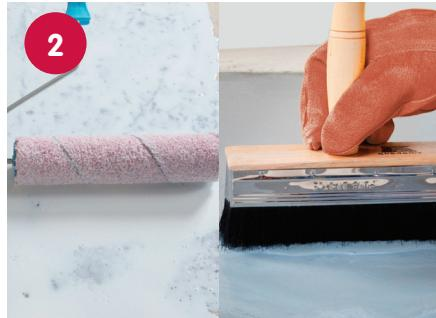
All substrates must be primed prior to the TAL Superflex application. Prime woodfloated substrates with TAL Floor Primer and powerfloated / steelfloated surfaces with a TAL Floorkey Slurry.
