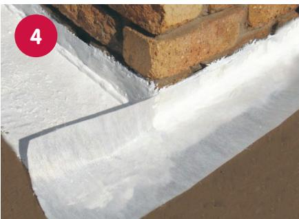
Apply a coat of TAL Superflex by brush or roller to the interfaces. Immediately bed a 200mm wide strip of TAL Superflex Membrane into the wet TAL Superflex, with the membrane extended 100mm on either side of the interface.
