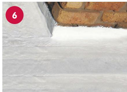
It is essential that the main TAL Superflex application overlaps the corner joints, i.e. the interface application must be completely covered by the main area application.
