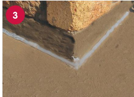
To allow for movement a 10mm bead of flexible silicone must be applied into all internal corners and interfaces prior to the TAL Superflex application.
