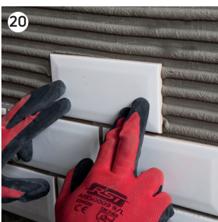
20 If tiling use a quick or rapid setting adhesive replace the water with TAL BOND. Then use TAL grout mixed with TAL BOND to finish the installation.
