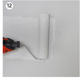
12 Apply the second coat in a horizontal direction to the first coat to ensure complete coverage and no pinholes.
