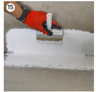
15 Apply a coat of TAL SUPERFLEX FIBRE 1K by brush.
