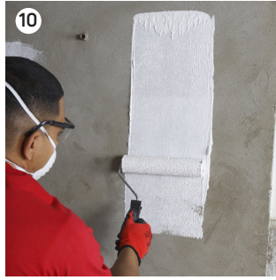
10 Apply the first coat to the clean dry surface with a short pile mohair roller in a vertical direction
