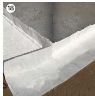
18 Ensure that the main area application overlaps the Interface applications.
