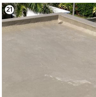
21 TAL SUPERFLEX FIBRE 1K can be left exposed on non-trafficable roof slabs and parapet walls.
