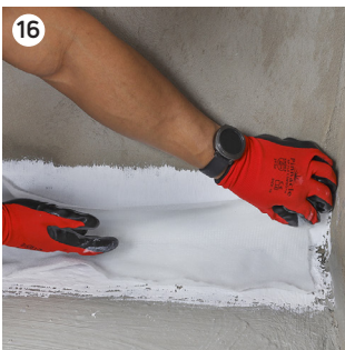
16 Immediately bed the TAL SUPERFLEX MEMBRANE into the wet coat.
