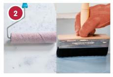
The substrate to be waterproofed must be clean, dry, firm and sound, free from dust, loose particles and surface contaminants, and must have a moisture content of less than 5% before the waterproofing can be applied. All substrates must be primed prior to the TAL Sureproof application - woodfloated surfaces with TAL Floor Primer and powerfloated / steelfloated surfaces with a TAL Floorkey Slurry.
