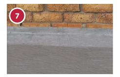
It is essential to ensure that the main TAL Sureproof application overlaps the corner joints/interfaces, i.e. the interface application must be completely covered by the main area application.
