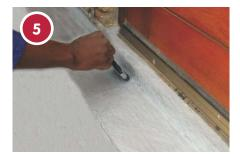
Apply a coat of TAL Sureproof by short hair enamel paint roller or brush to the interfaces. Immediately bed a 200mm wide strip of TAL Sureproof Membrane into the wet TAL Sureproof, with the membrane extended 100mm on either side of the interface. The membrane must be pushed into the corners. Apply a heavy topcoat of TAL Sureproof over the membrane to saturate the membrane before the first coat dries.
