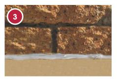
To allow for movement a 10mm bead of flexible silicone must be applied into all internal corners and interfaces prior to the TAL Sureproof application.
